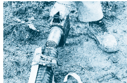
3. Use hot air or hot water to heat the medium pipe; let it cool – and the job is finished.
