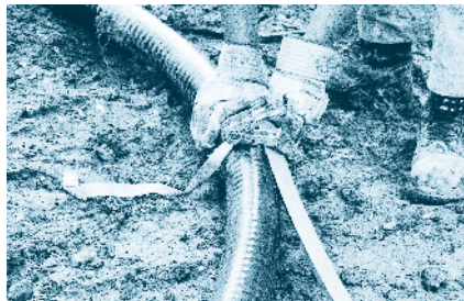
1. Fix the CALPEX-pipe to one end of the rail, using the tensioning belt.
