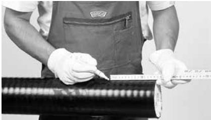
1 Mark the distance (x, y, z) + 1 cm from the end of the pipe.
