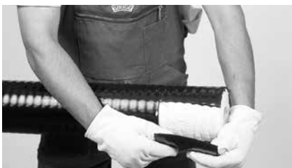
4 Peel off the casing.
