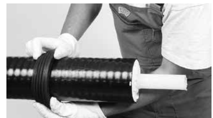
6 Install the wall sealing ring.
