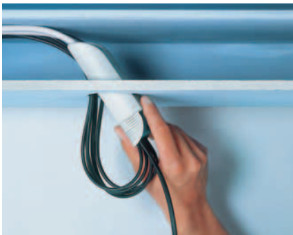
The wired 150 W Mouse is inserted in the opening with the primary side first.
