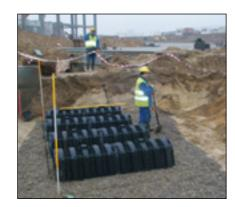
**Stormwater management ►** Infiltration Tunnel / twin
